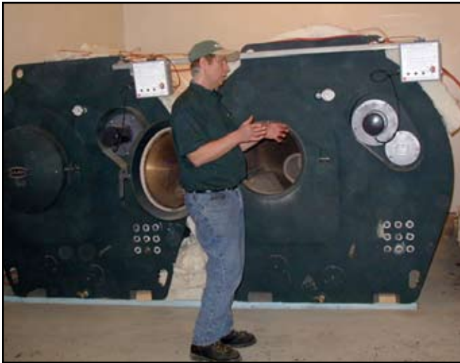
Above Left: Dave Frederick of Alaskan Heat Technologies explains the operation of GARN wood-fired boilers in Tanana, AK. Photo by Daniel Parrent
